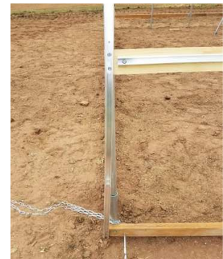
Figure 27 –U-Channel End Wall Attachment
