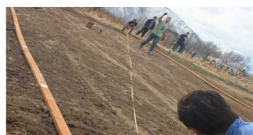
Figure 5 – Measuring diagonal corners
