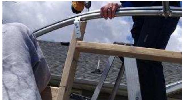
Figure 22 – Metal straps as seen from the inside of the hightunnel.
