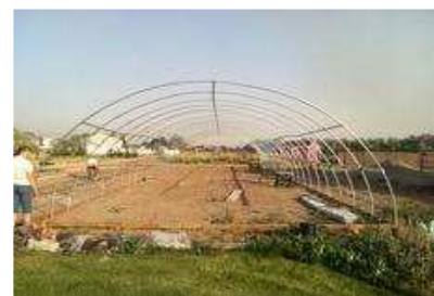
Figure 19 – Hightunnel with Purlins & Pipe finished
