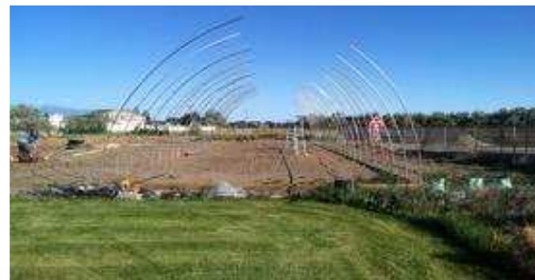
Figure 13 - Ribs hanging free waiting for joining
