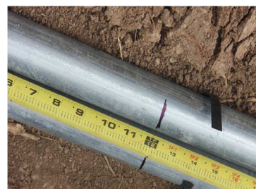
Figure 4 – 12” Marking on posts
