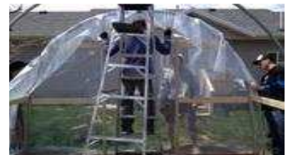
Figure 28 – Plastic on End-Wall
