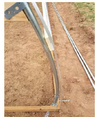
Figure 27 –U-Channel End Wall Attachment
