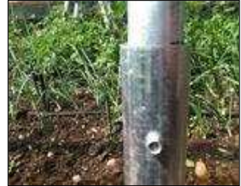
Figure 15 – Securing rib into post
