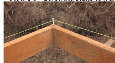
Figure 9 – Leveling base with the string
