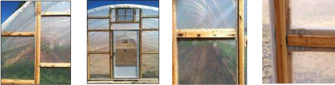
Figure 30 – Furring Strips on End Walls
