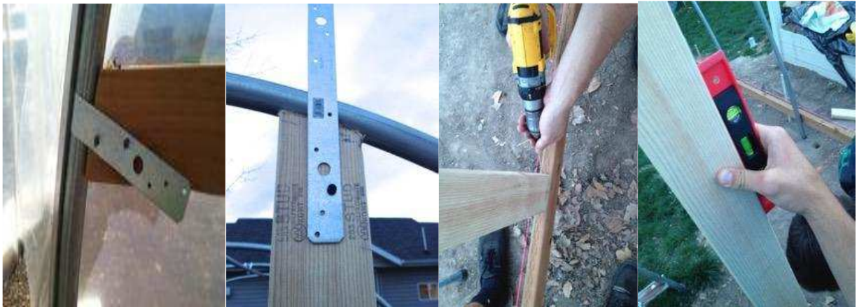
Figure 21 – Framing ends of hightunnel (Metal straps looking from the inside, on far left).
