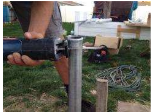
Figure 10 – Cutting off smashed post
