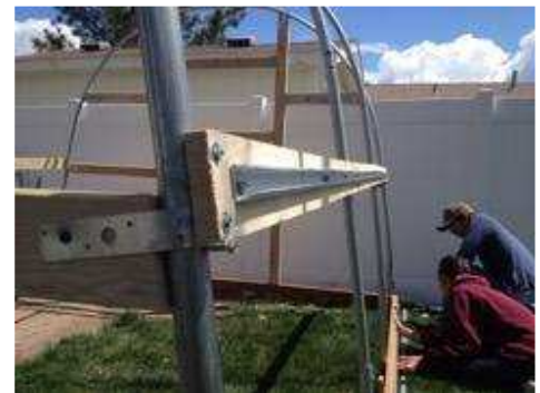
Figure 25 – Mounted Roll-Up Boards
