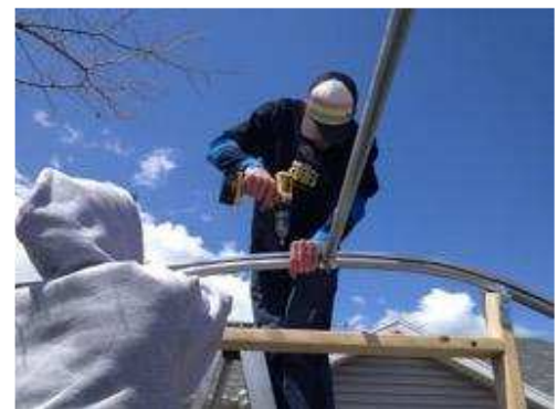
Figure 26 – Attaching U-Channel
