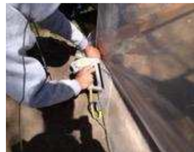
Figure 29 – Stapling the plastic to the frame
