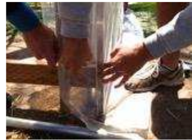
Figure 29 – Stapling the plastic to the frame
