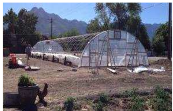
Figure 33 – Roll-Up Bars on the side of hightunnel
