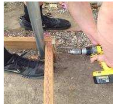
Figure 8 – Screwing stake to frame
